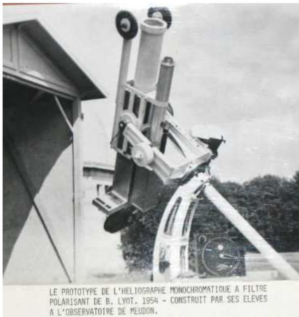
LE PROTOTYPE DE L'HELIOGRAPHE MONOCHROMATIQUE A FILTRE POLARISANT DE B. LYOT, 1954 - CONSTRUIT PAR SES ELEVES A L'OBSERVATOIRE DE MEUDON.
